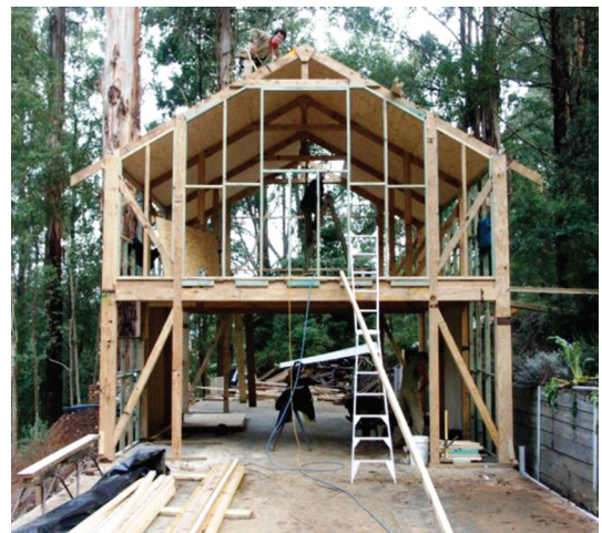
Standard Module: 7.2m x 6.0m = 40m 2 upper floor and 43m 2 ground floor area
